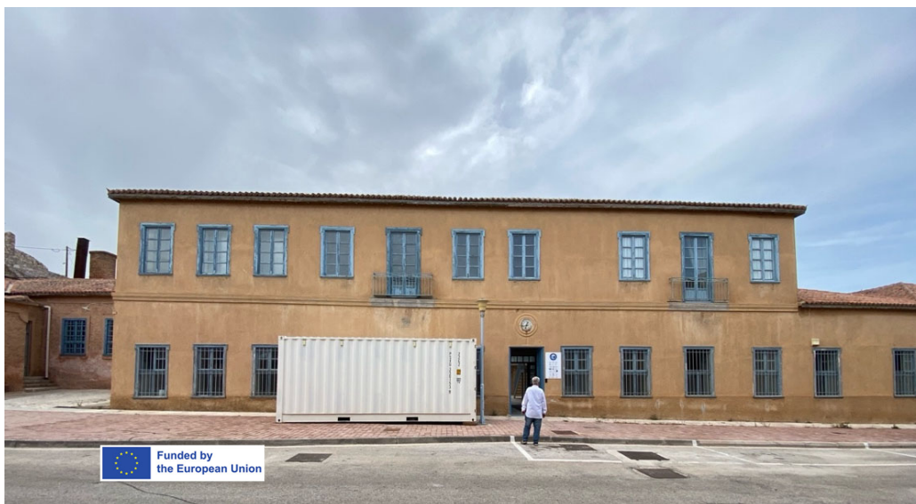
Figure 1. The 'Robot Cabin,' deployed by TSIKIS within a white LR-certified ISO 6-meter open-side container, situated at the Lavrion Technological and Cultural Park next to the 'ROLOI' Building.
